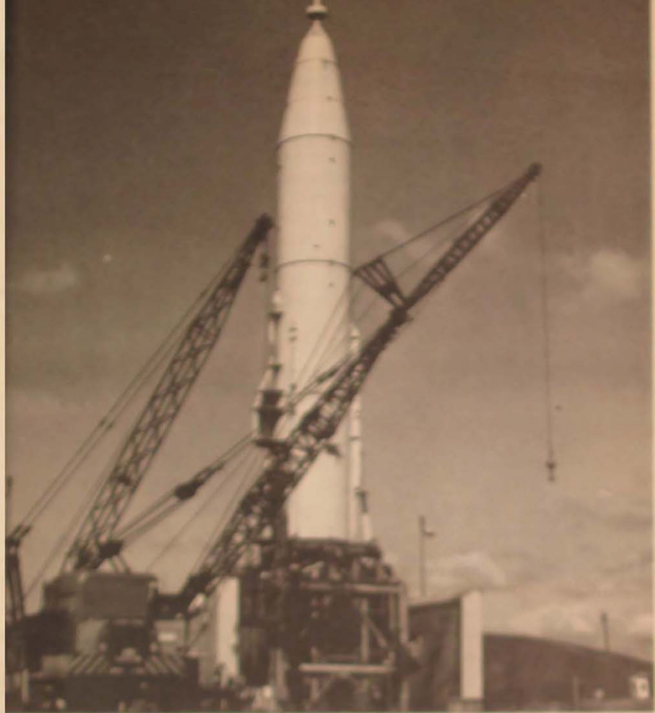
The "Water Bird" test tool, used in activation-verification exercises at Vandenberg AFB, helps test the Atlas F launch platform lifting system. Weight of the tool-apt, which is built to scale, is varied by the amount of water pumped into it.
