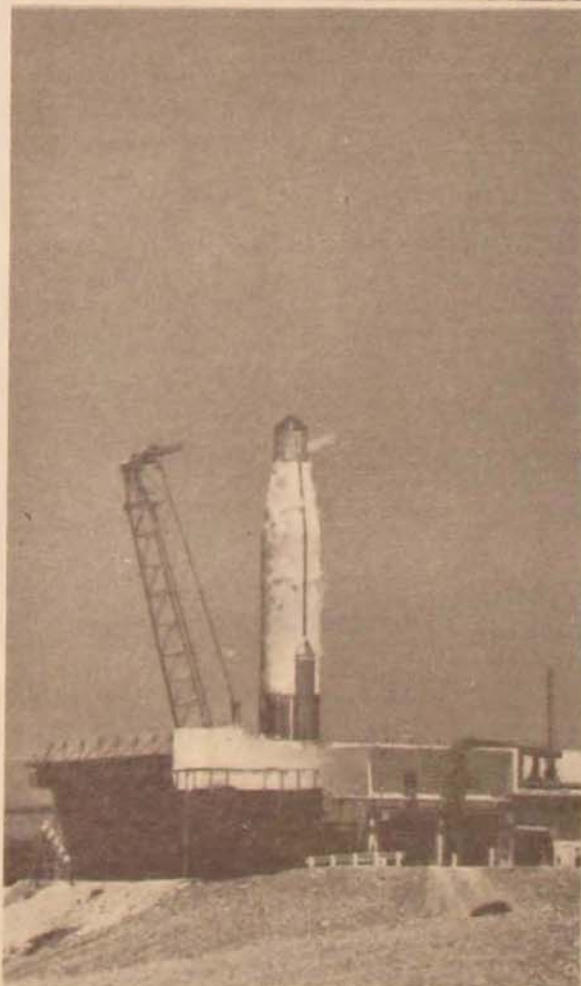
Reaction capability of the Atlas in launch from the semihard or "coffin" emplacement is shown in sequential photographs taken during the 15-minute period of a training launch conducted at Vandenberg AFB, California. The flight was
