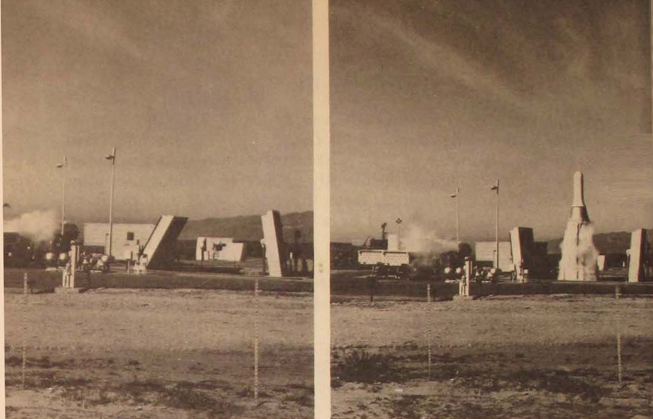
The missile used for initial chilling tests on the Atlas F silo test facility never leaves the launch, but it does simulate all prelaunch missile functions. Liquid
